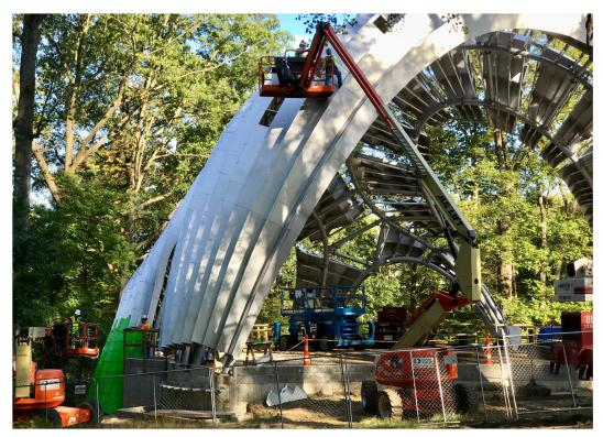
On top of the ZEPPS (which are composed of 300 unique aluminum trusses), clear anodized aluminum sheeting is secured, forming the silver colored, exterior substrate and interior finished surface geometry of the Chrysalis' highly functional sculpture. While the last of this aluminum sheeting is screwed into the ZEPPS, the outer layer of 7,700 colored shingles is carefully attached. The shingles come in 11 sizes and shapes, and in four different shades of <u>Spring Green</u>.
