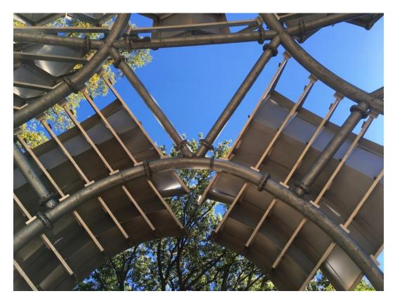
On top of the double curved, tubular, galvanized steel frame, <u>Zahner</u> has designed, engineered, fabricated, and is erecting and installing the Chrysalis' 12,000 square feet of aluminum skin. More than seventy five (75) <u>ZEPPS</u> (<u>Zahner Engineered</u> <u>Profiled Panel Systems</u>) define the structural geometry and surface of the skin, each about the size of a small car.
